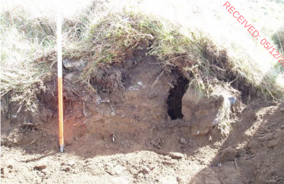
Fig. 14. Cutting 2a Section of field boundary looking north
